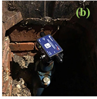
Fig. 5: Place an acceleration on gate valve[17]
